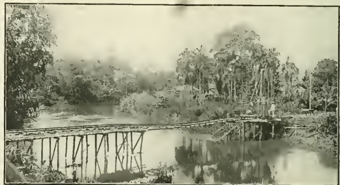
TRESTLE BRIDGE WITH SUPPORTS WASHED OUT.
